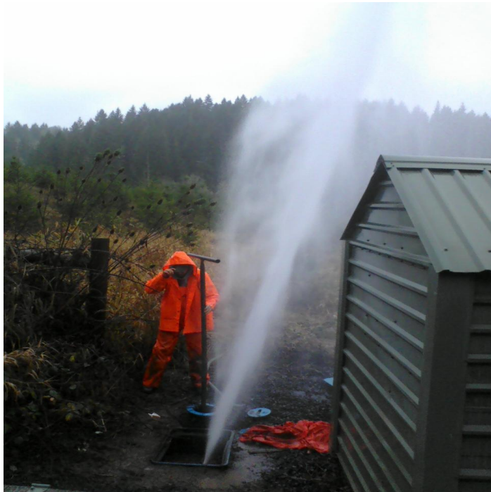
Water shooting out of the ground
